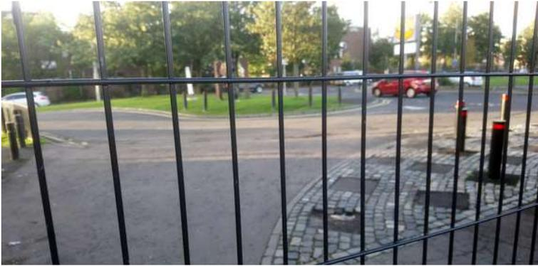
In order to prevent damage from strong wind, the cladding on the staff and traders' car park gate was changed from solid steel sheeting to 'paladin' type steel mesh. The effect of this has been to change the nature of the interface at this location such that some housing within Suffolk estate can now be seen from the Stewartstown
